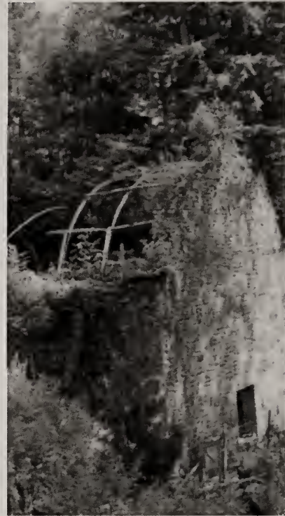
The derelict fernery with its towering south gable.
