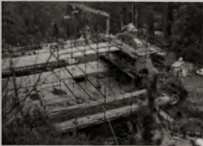
Above: Work in progress.
